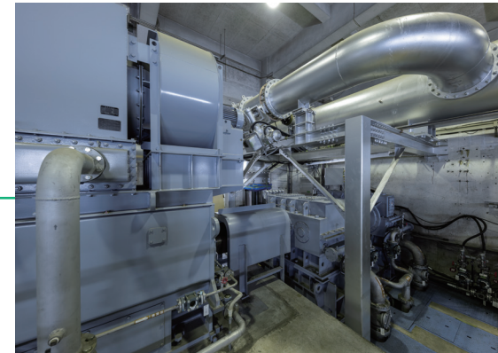
8MW系駆動装置 Electric Motor and Gear Box for High-Pressure Test Rig
