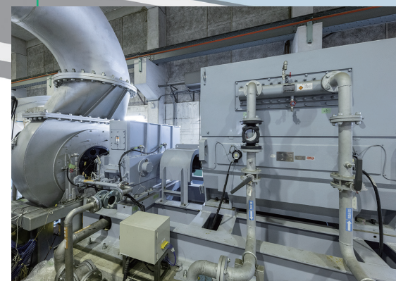
2.2MW系駆動装置 Electric Motor and Gear Box for Low-Pressure Test Rig
