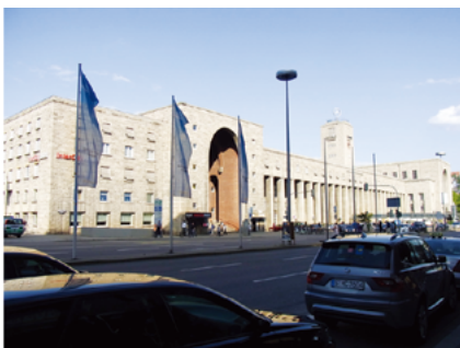
Station where reconstruction has begun
